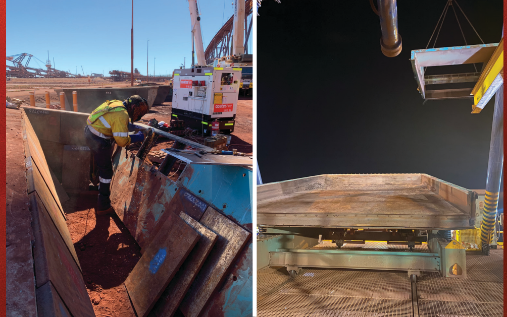
Project: Replace Hopper Liners
