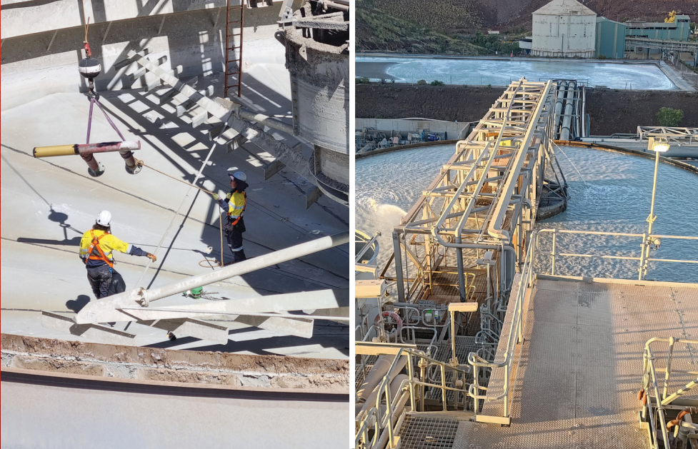
Project: Inspect, Report & Repair Tank
